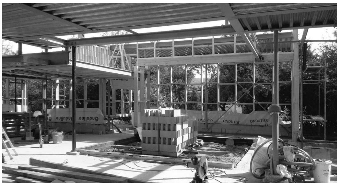
*Structure poteaux-poutres et plancher collaborant*
