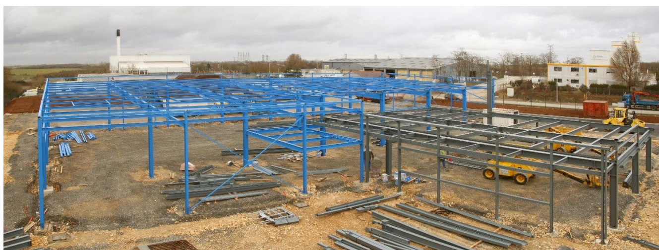
Portiques plan (Hall) ossature poteaux-poutres (Bureaux)
