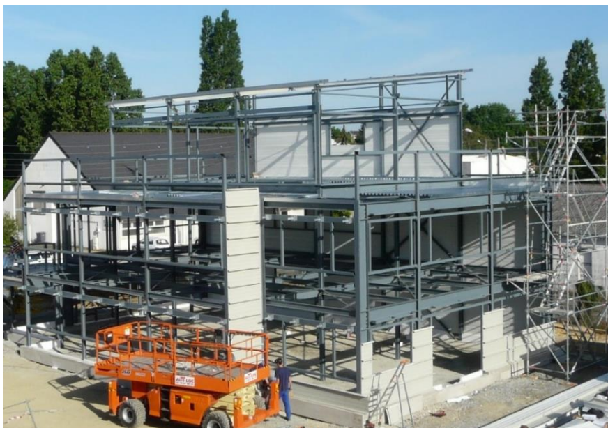
Ossature poteaux-poutres multi-étages
